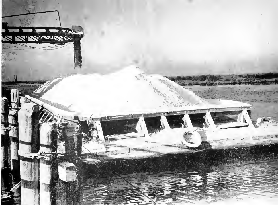
Loading Sulphur on Barge, Grande Ecaille, Louisiana.
